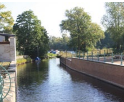
Second construction phase of the city canal at street 'Heilig-Geist-Straße' (75)
