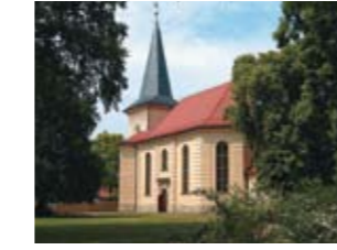
Friedrich Church near Weberplatz (14)
